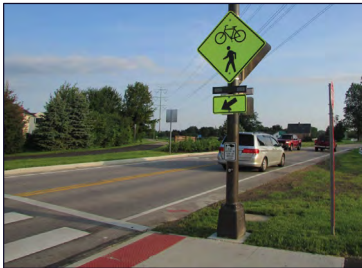
Figure 12 – Example of RRFB 4
