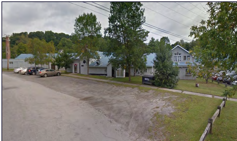
Figure 21 – Existing sidewalk in the Valley Bowl Complex 15
