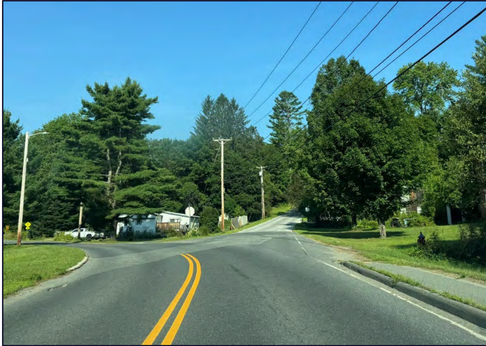
Figure 29 – View of current VT12A / Wallace Hill Rd intersection
