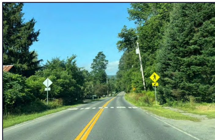
Figure 11 – View of crosswalk on Park Street (VT12A) to Recreation Fields
