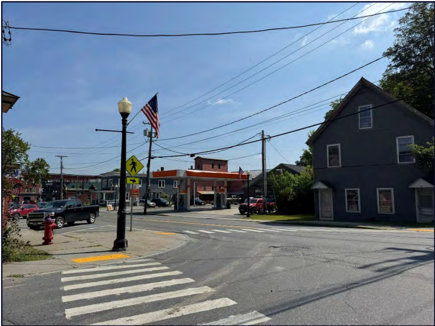
Figure 10 – View of crosswalk and obscured sight distance of vehicles traveling southbound
